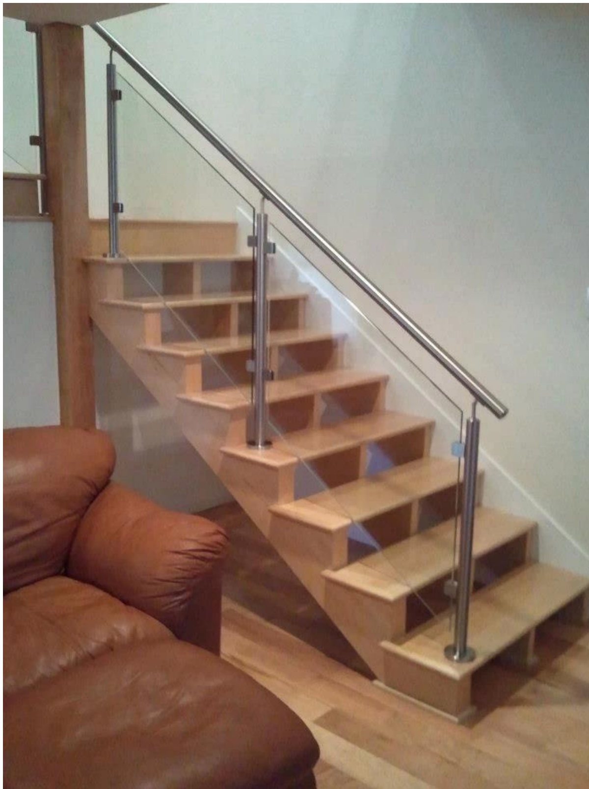
Staircase with wooden steps, stainless steel handrails, and glass railing. A brown leather sofa is visible in the foreground.
