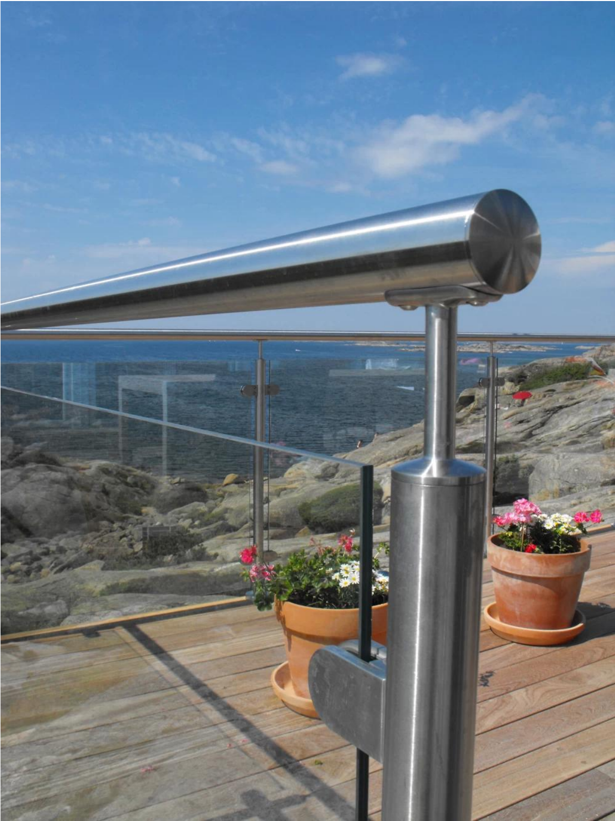
Figure 1: A stainless steel railing system installed on a wooden deck overlooking a rocky coastline and the ocean. The railing features a thick horizontal top rail supported by vertical posts. Two terracotta pots with pink and white flowers are placed on the deck. The background shows a clear blue sky with light clouds.
