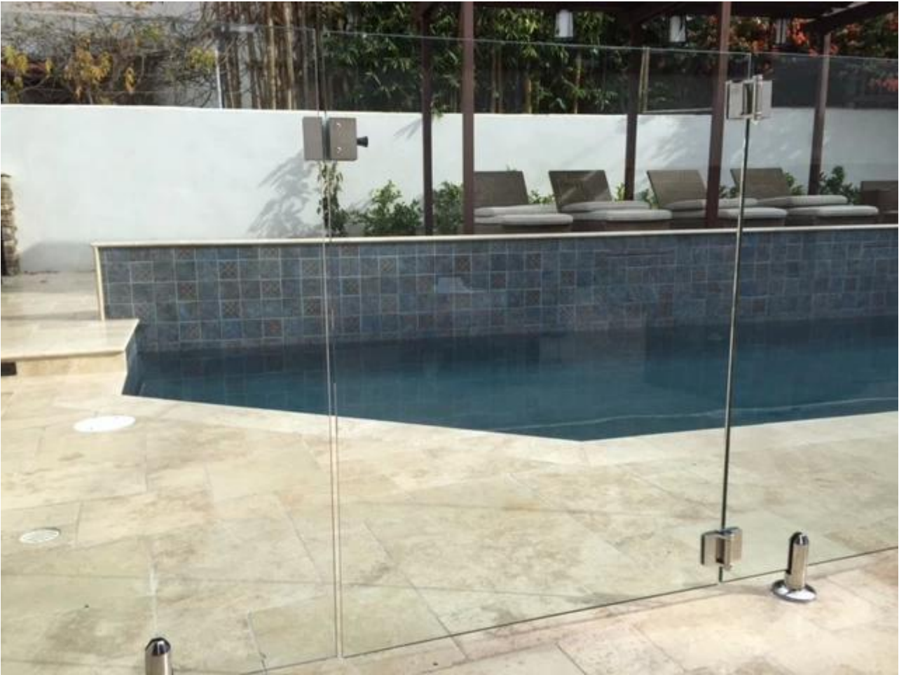
G-G1: sheet metal glass to glass hinge
