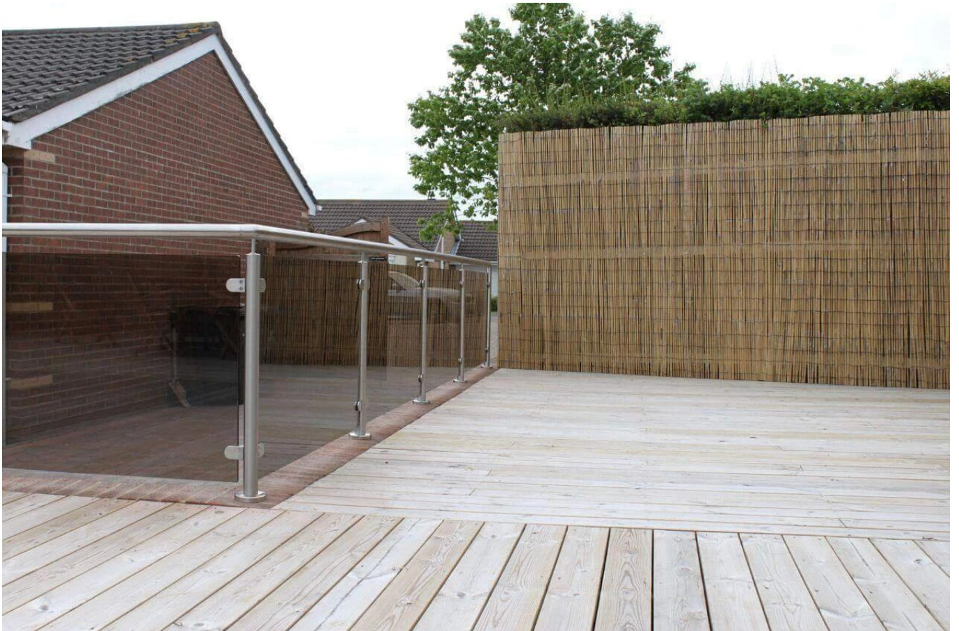
# Installation photos of stainless steel post handrail bracket
