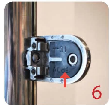
Select appropriate rubber gasket to suit glass panel thickness. Install rubber gasket into both sides of glass clamp. (Note rubber gasket marked with sizes).
