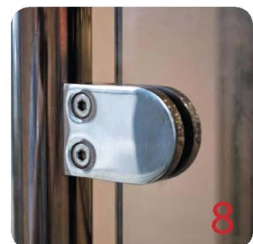
Tighten glass clamps with hex key, and check glass panel are secure with no movement.
