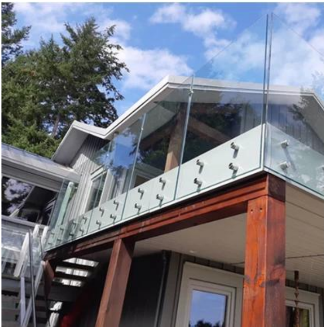
2" Diameter Glass Clamps Standoff for Mounting to Wooden Substrate:
