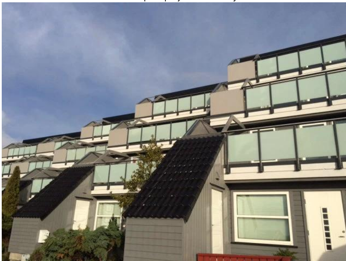
Side mounted aluminum handrail post project in Norway
