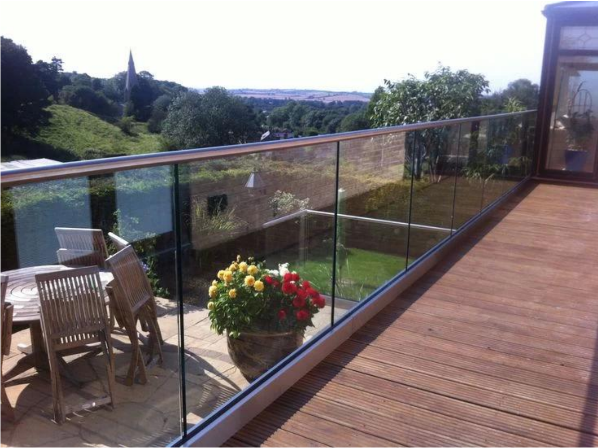
Aluminum U channel + 10-12mm tempered glass design
