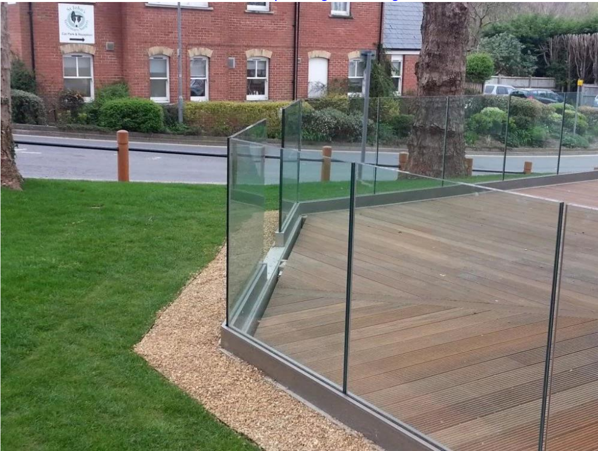
Aluminum U channel + 10-12mm tempered glass design
