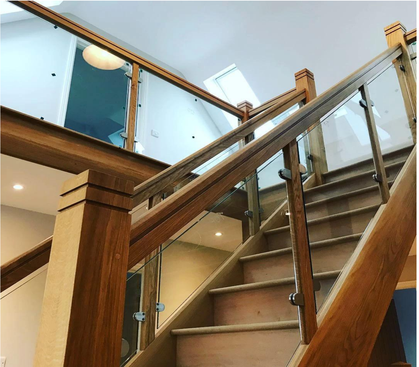
The glass railing clamp usually used with stainless steel post to hold glass panels, for balcony railing, terrace railing, staircase. Suitable for both indoor and out door.
