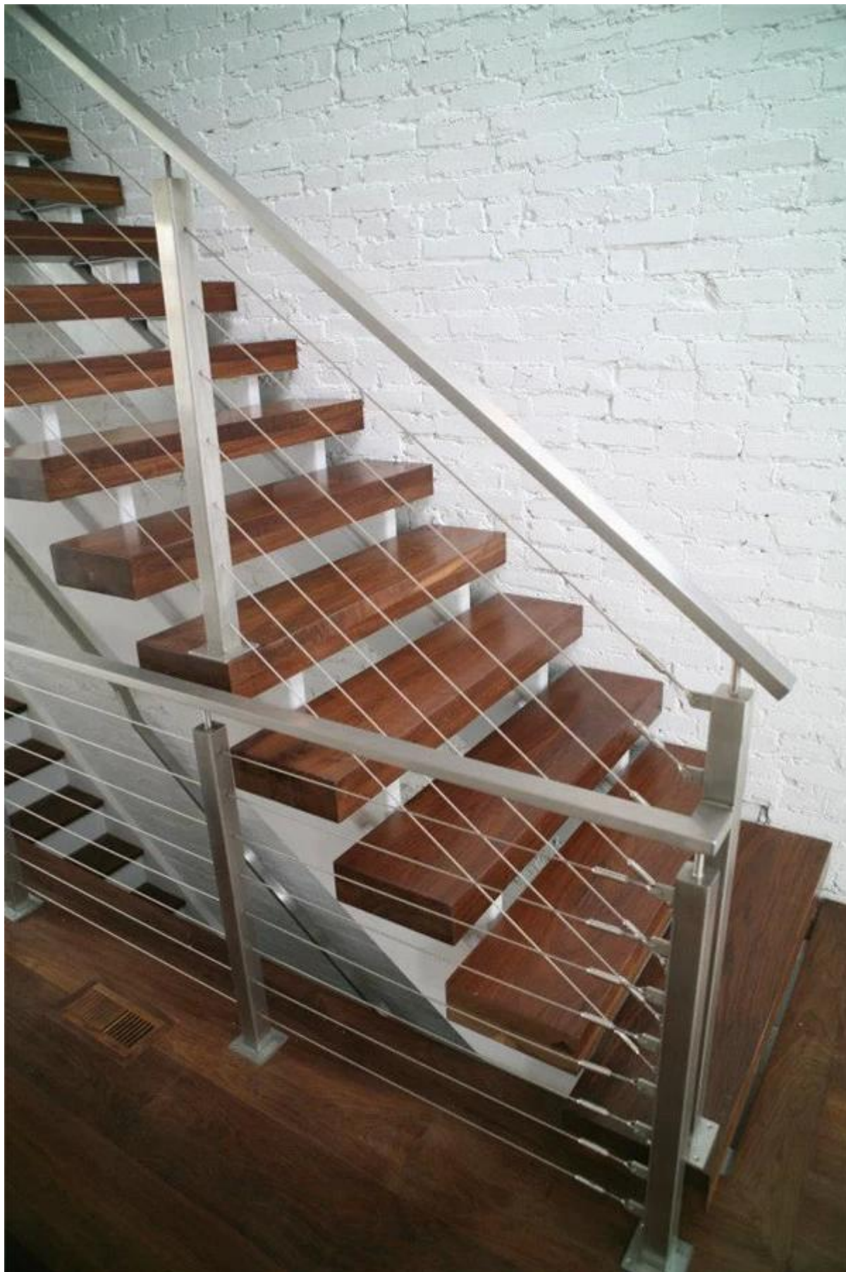
Model No.: LCH-124 material: stainless steel 304/316
