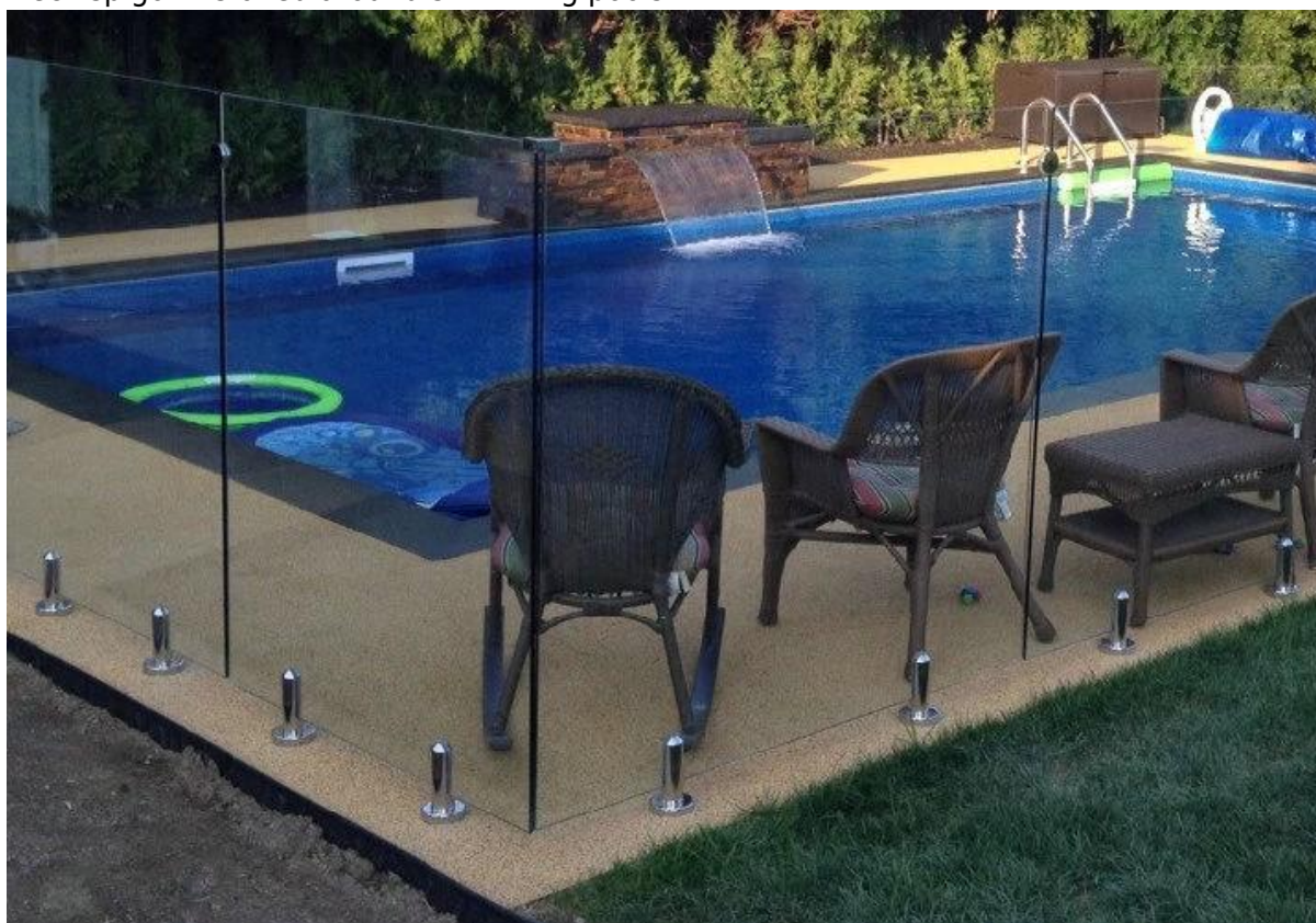
Deck spigot installed around swimming pools :
