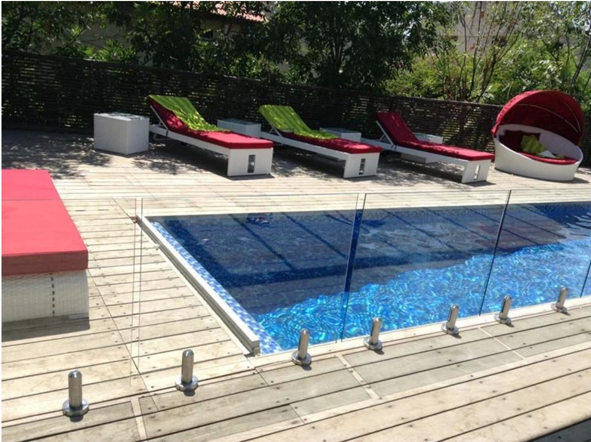
frameless glass railing with spigot
