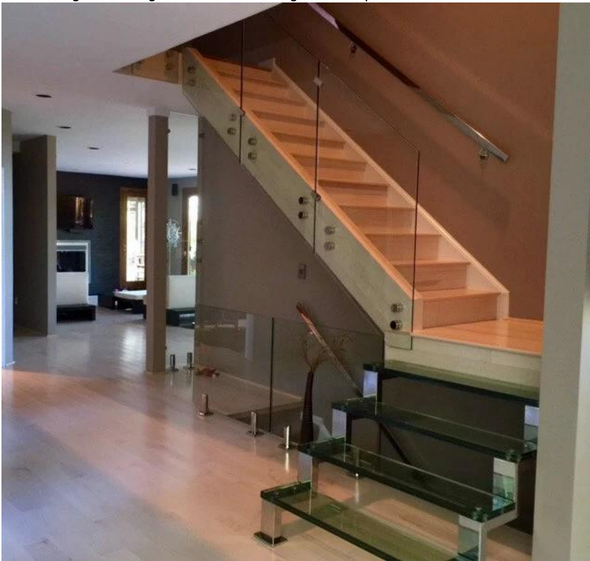
Staircase glass railing with standoff and glass clamp
