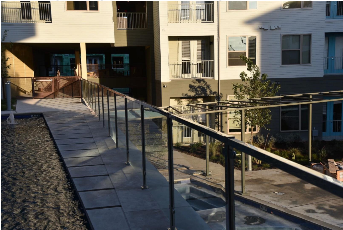
3. Installation photos of square 80x80mm stainless steel post with sealed end cap
