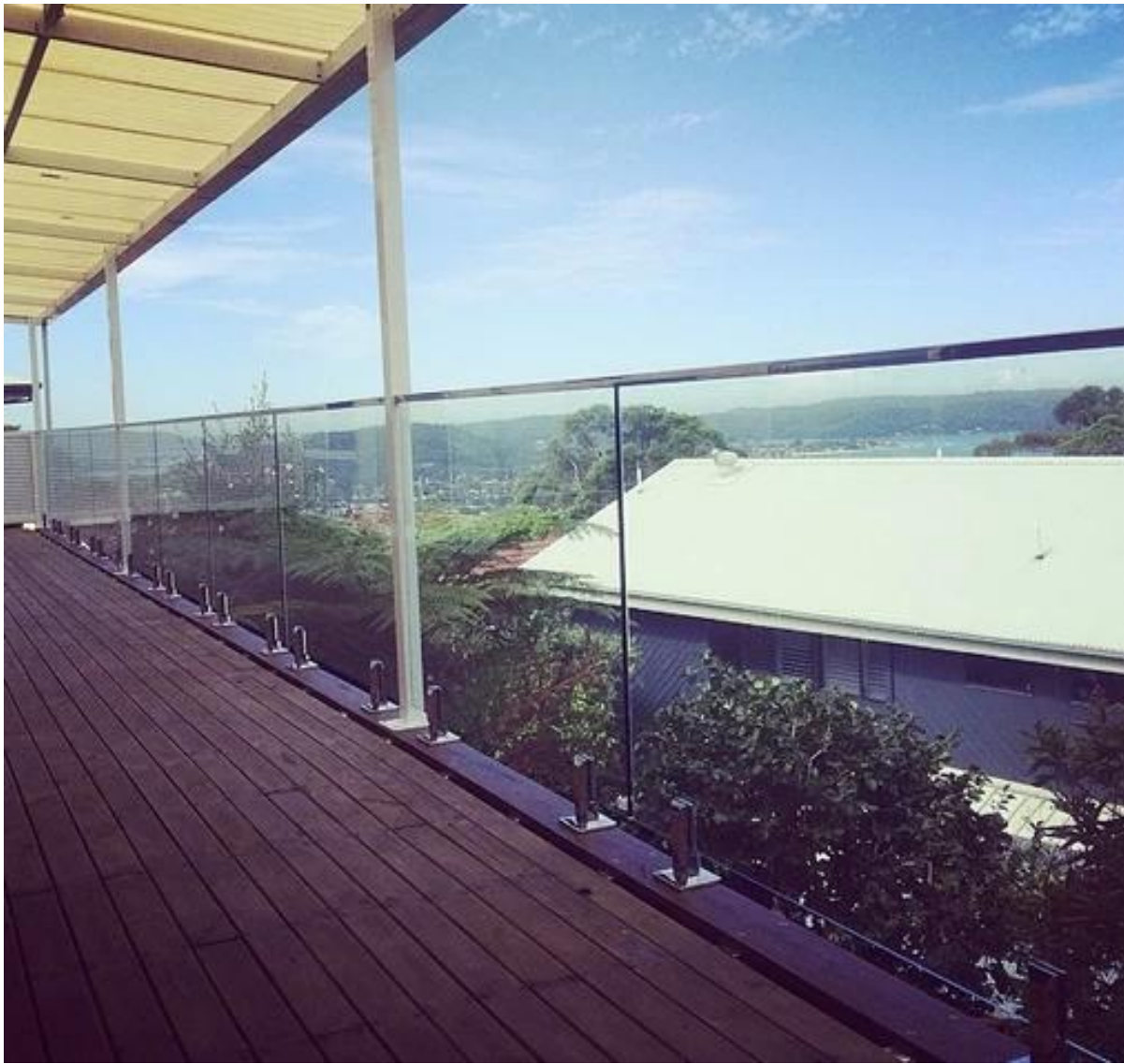
4. Round shape diameter 25.4mm stainless steel balustrades top rails.
