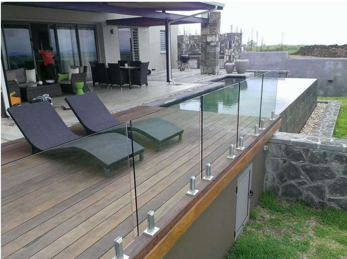
4. 4 types stainless steel spigots,
