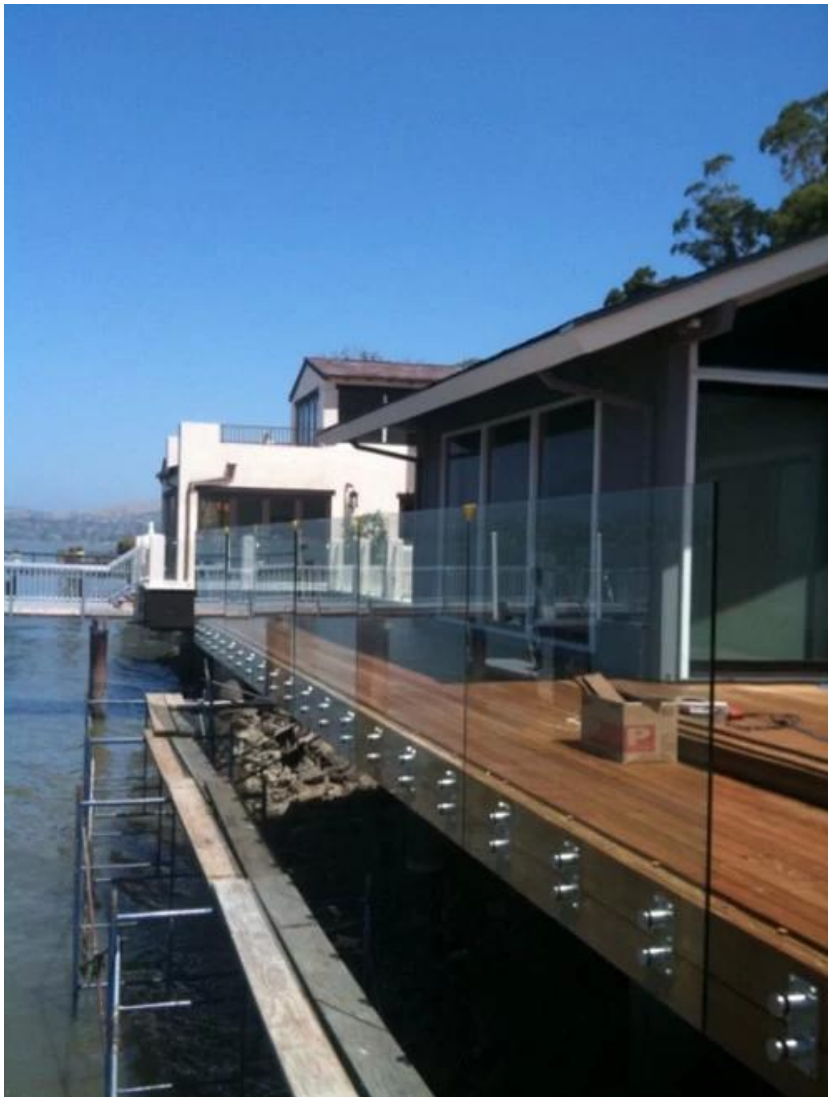
deck mount, stainless steel square spigot, pool fencing or balcony railing
