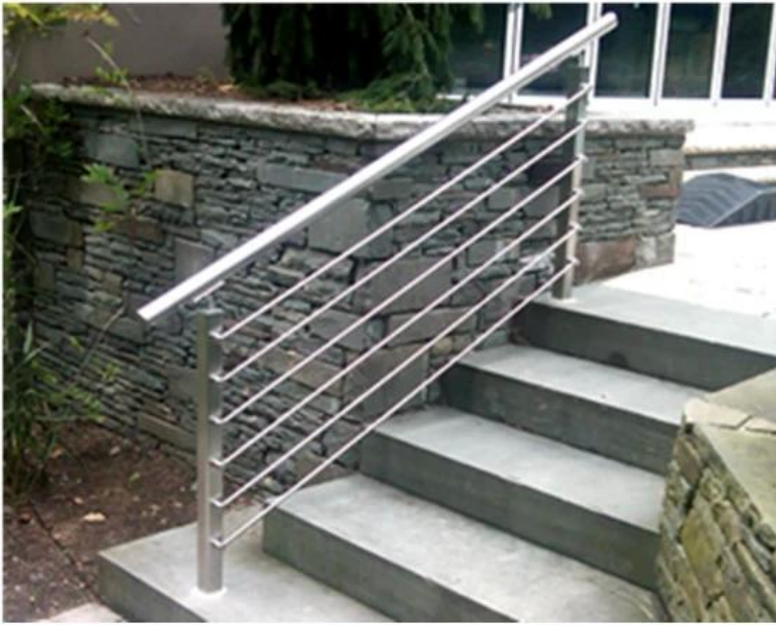
stainless steel handrail with cross bar
