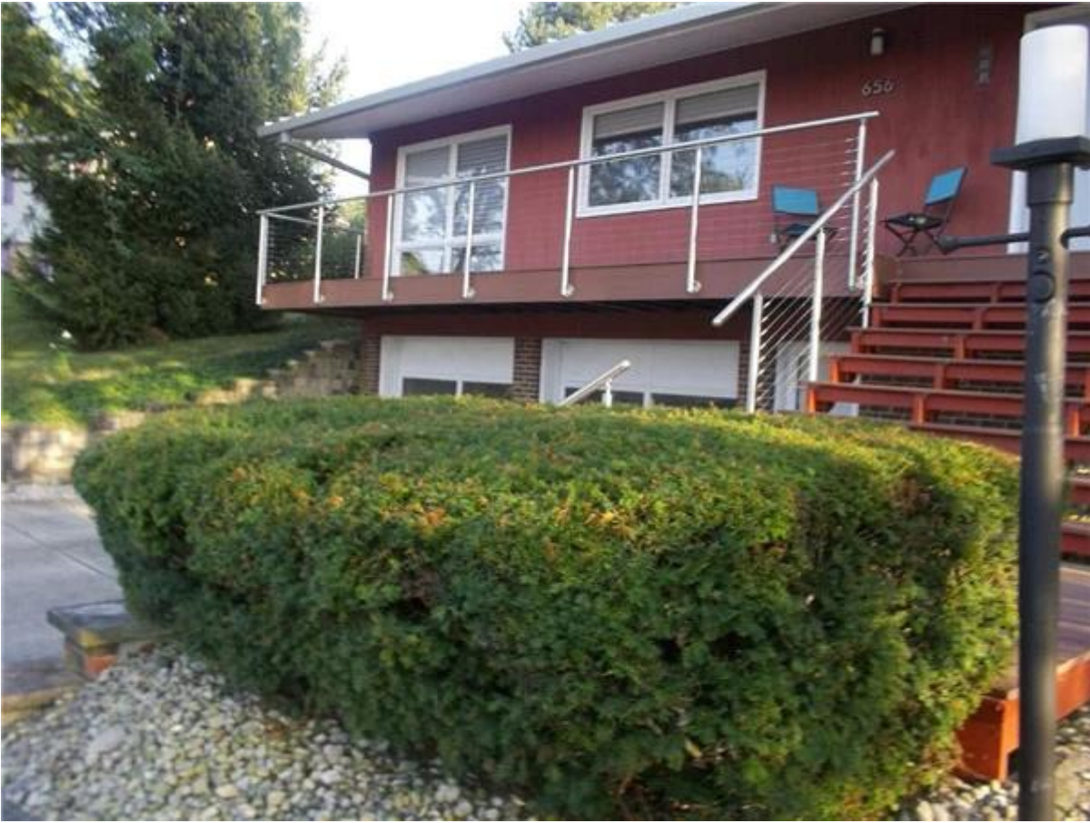
2. Photos of wire rope railing posts-
