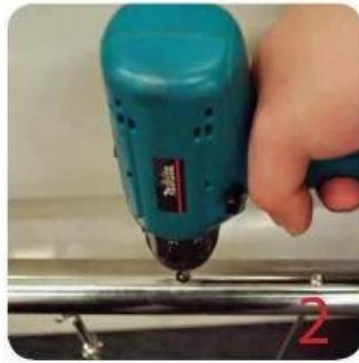
Drill centre punched hole in tube to suit blind rivet nut.
