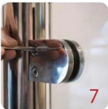
Fit glass panel into position, install second half of glass clamp secure with provided hex screws.
