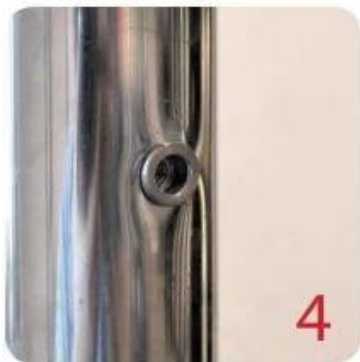
Check installed blind rivet nut is secure and ready for install.
