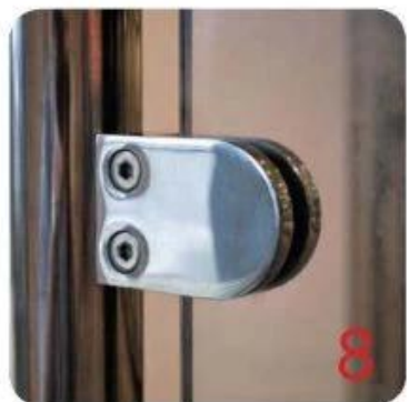
Tighten glass clamps with hex key, and check glass panel are secure with no movement.
