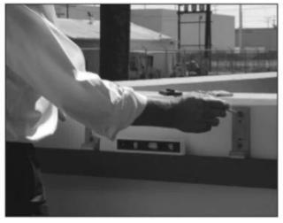
With the front face plate removed, level or align the Clamps to your design plan, taking into account the spacing recommendations and weight limitations shown on the back of this page. Be sure to secure the Clamps to an engineered and approved substrate with appropriate fasteners. You can fabricate the glass ahead of time, however, we recommend calculating hole locations after the Clamps are installed to account for any clamp movement.
