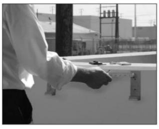
Check the layout of the Clamps for alignment, then do a layout for fabricating holes in the glass to meet the installed measurements and spacing between glass panels.
