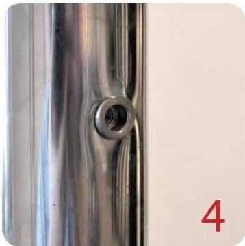
4 Check installed blind rivet nut is secure and ready for install.
