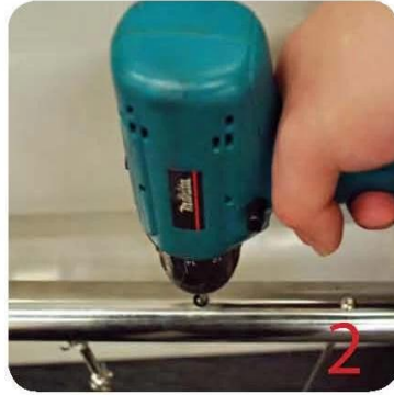
2 Drill centre punched hole in tube to suit blind rivet nut.
