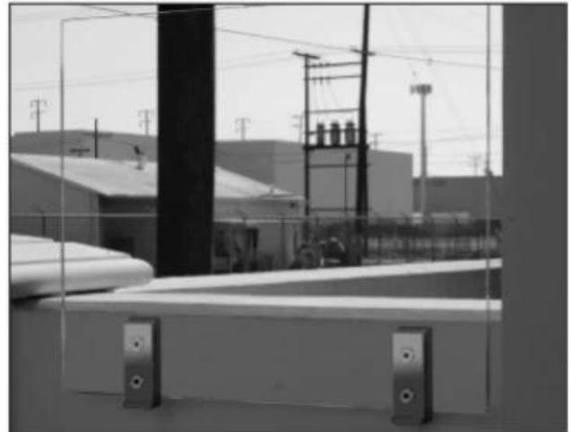
After you have achieved the proper alignment tightly secure the front plate screws to finish the installation. Clean the glass and view from a distance to determine if everything matches up and looks good. Adjust if necessary.
