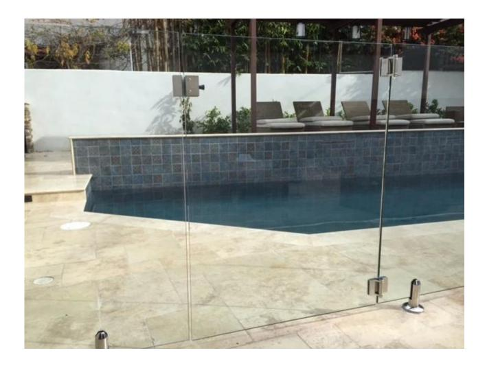
Model No.: G-G2(casting glass to glass hinge) material: stainless steel 316 finish: mirror or satin polished for glass thickness: 8mm
