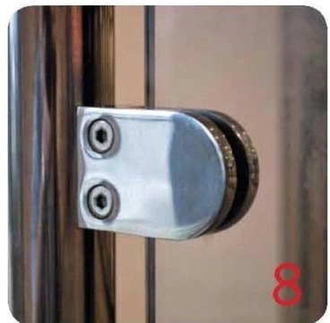
8 Tighten glass clamps with hex key, and check glass panel are secure with no movement.
