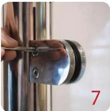
7 Fit glass panel into position, install second half of glass clamp secure with provided hex screws.
