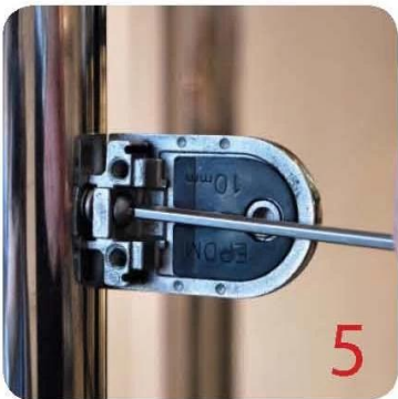
5 Align half glass clamp with blind rivet nut inline position. Screw in button head cap screw into thread and tighten with hex key.
