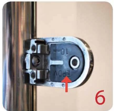
6 Select appropriate rubber gasket to suit glass panel thickness. Install rubber gasket into both sides of glass clamp. (Note rubber gasket marked with sizes).
