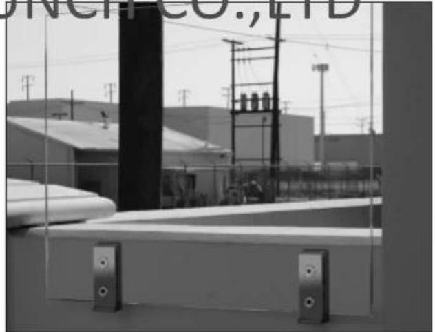
After you have achieved the proper alignment tightly secure the front plate screws to finish the installation. Clean the glass and view from a distance to determine if everything matches up and looks good. Adjust if necessary.
