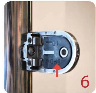
6 Select appropriate rubber gasket to suit glass panel thickness. Install rubber gasket into both sides of glass clamp. (Note rubber gasket marked with sizes).
