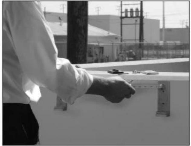
Check the layout of the Clamps for alignment, then do a layout for fabricating holes in the glass to meet the installed measurements and spacing between glass panels.
