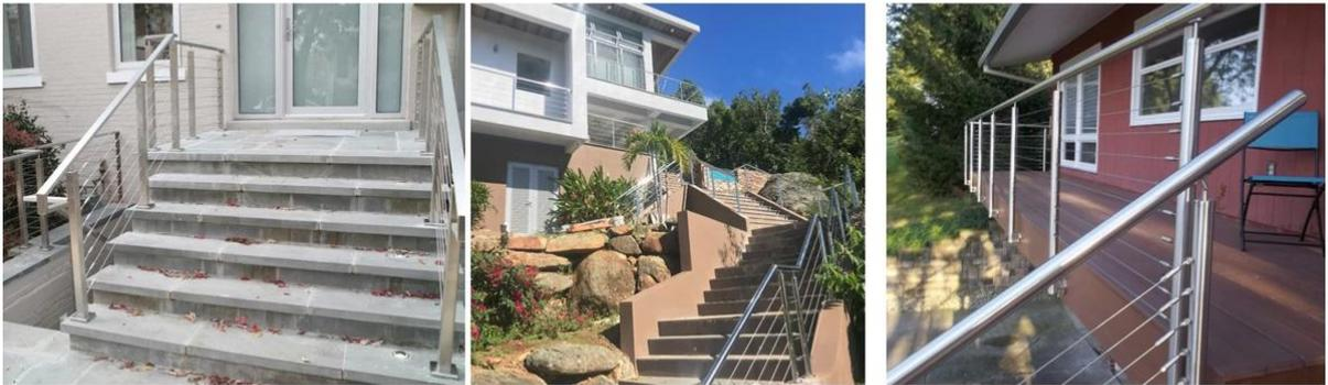
• 316 grade stainless steel exterior balcony and stair cable railings
