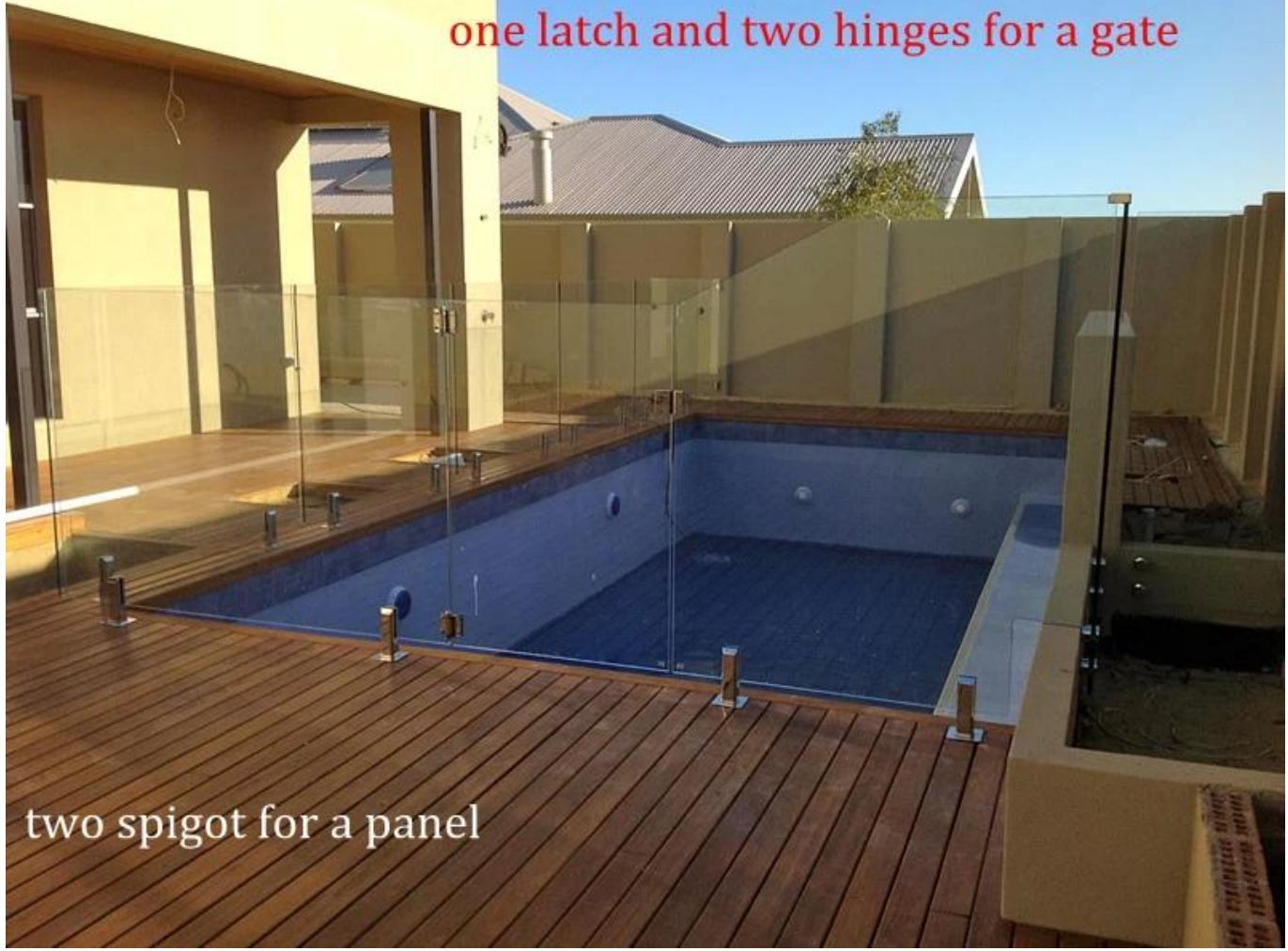
one latch and two hinges for a gate
