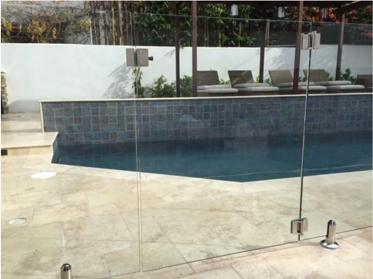
G-G1: sheet metal glass to glass hinge
