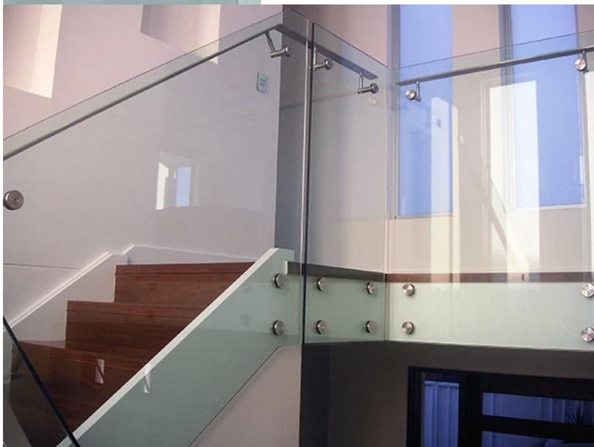
Frameloze glazen balustrade glas standoff pin
