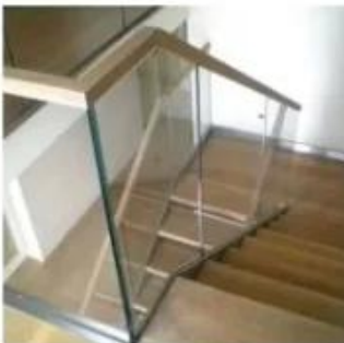
U channel glass railing
