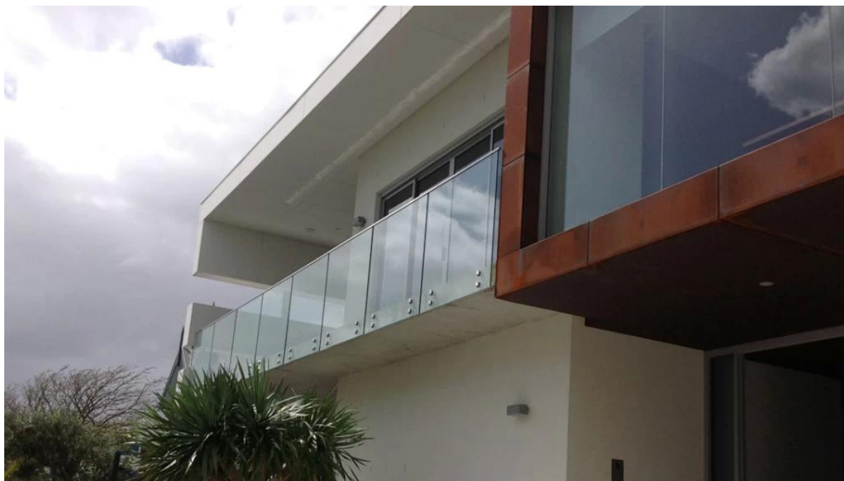
glazen trap RVS 316 massief glas standoff, buitenteras glazen balustrade project,
