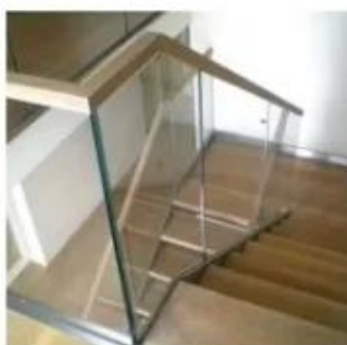
U channel glass railing
