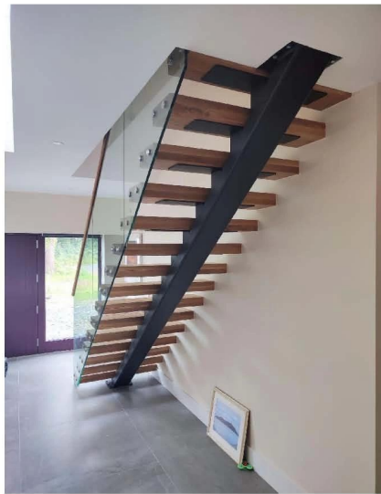
单龙骨楼梯 Mono Stringer stairs • Ireland stair 玻璃护栏 Glass railing
