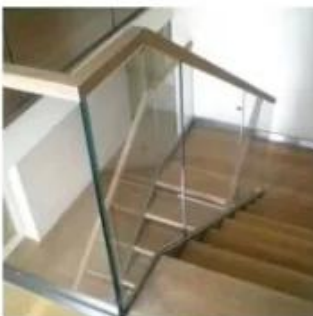
U channel glass railing
