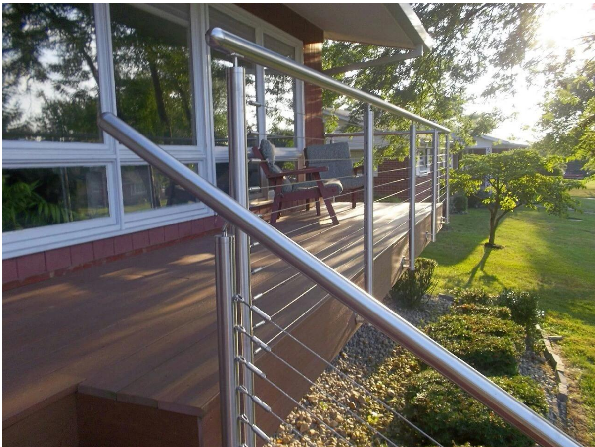
T803 mount to stainless steel post
