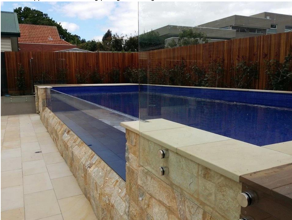
Standoff applied on swimming pool glass railings :
