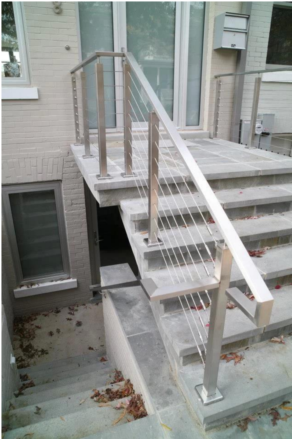
Fittings needed for square cable railing Square post
