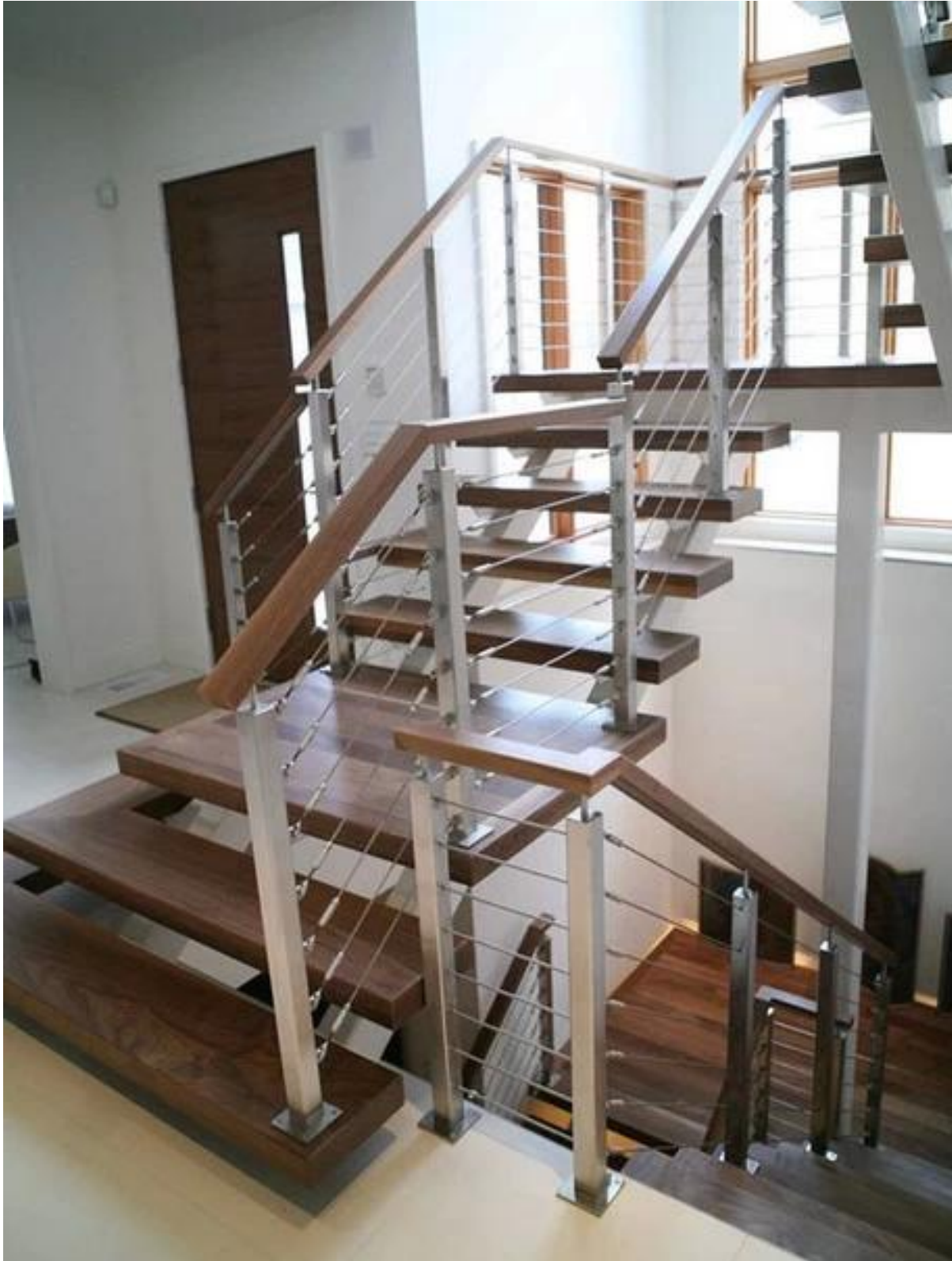
stainless steel railing string cable railig for stairs
