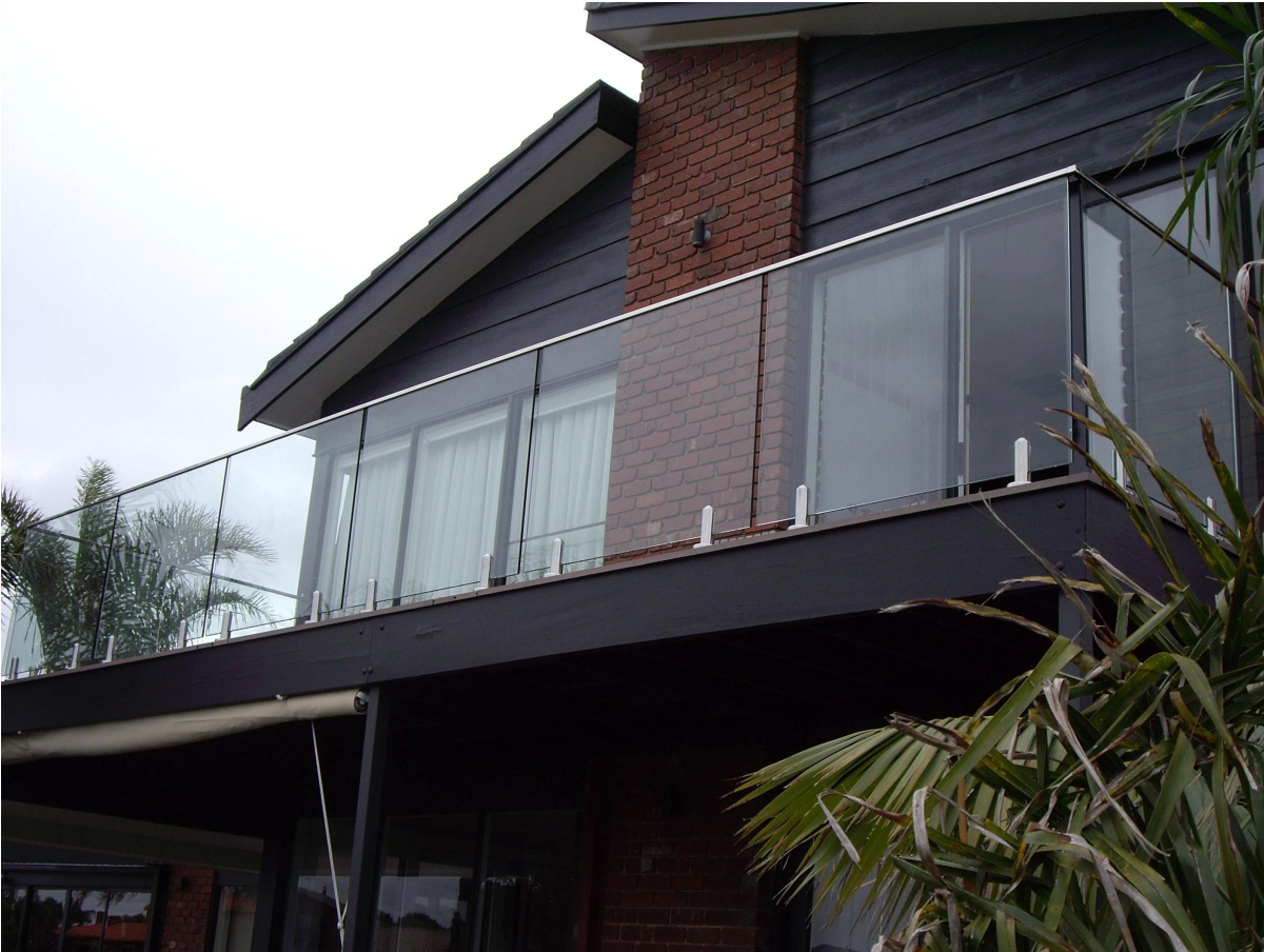
installation photo of 316 stainless steel slot top handrail 21x25mm indoors
