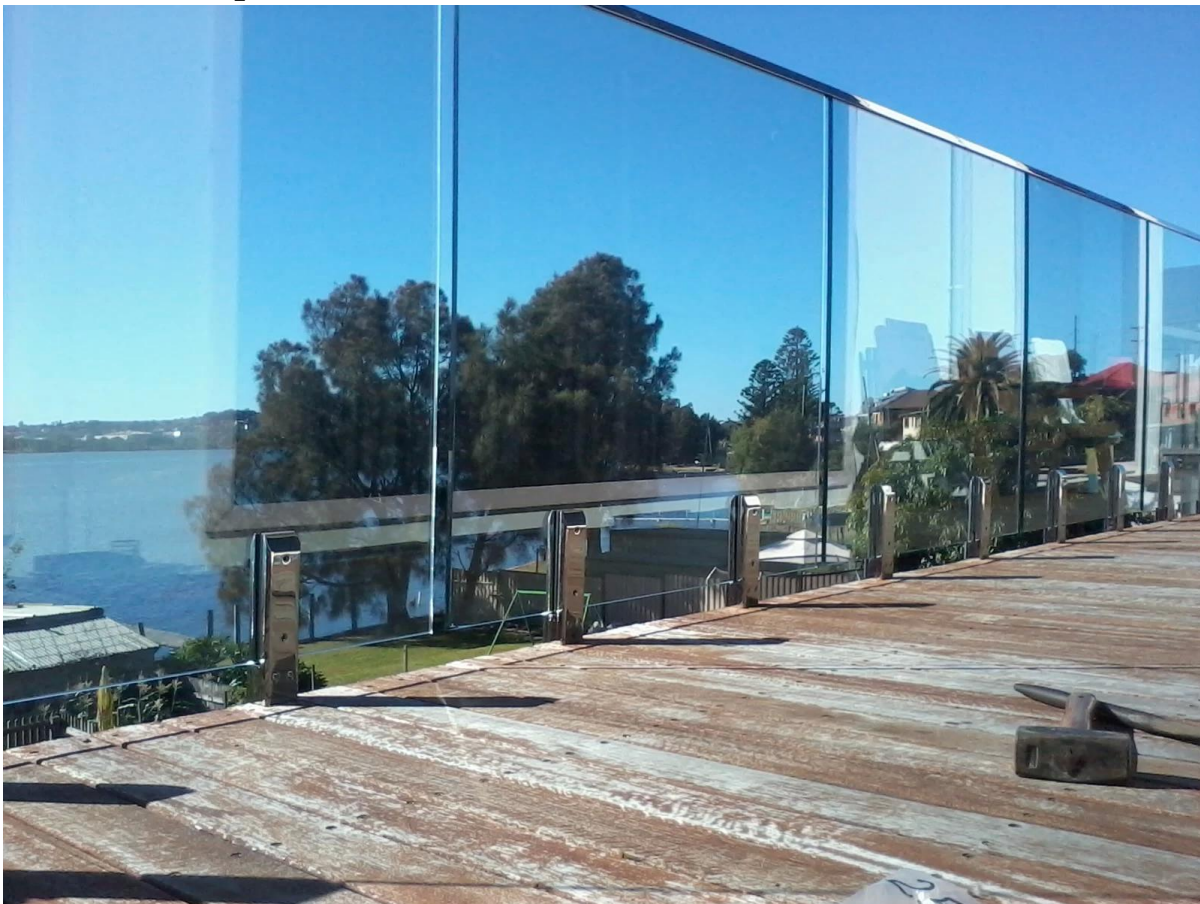
installation photos of slot handrails
