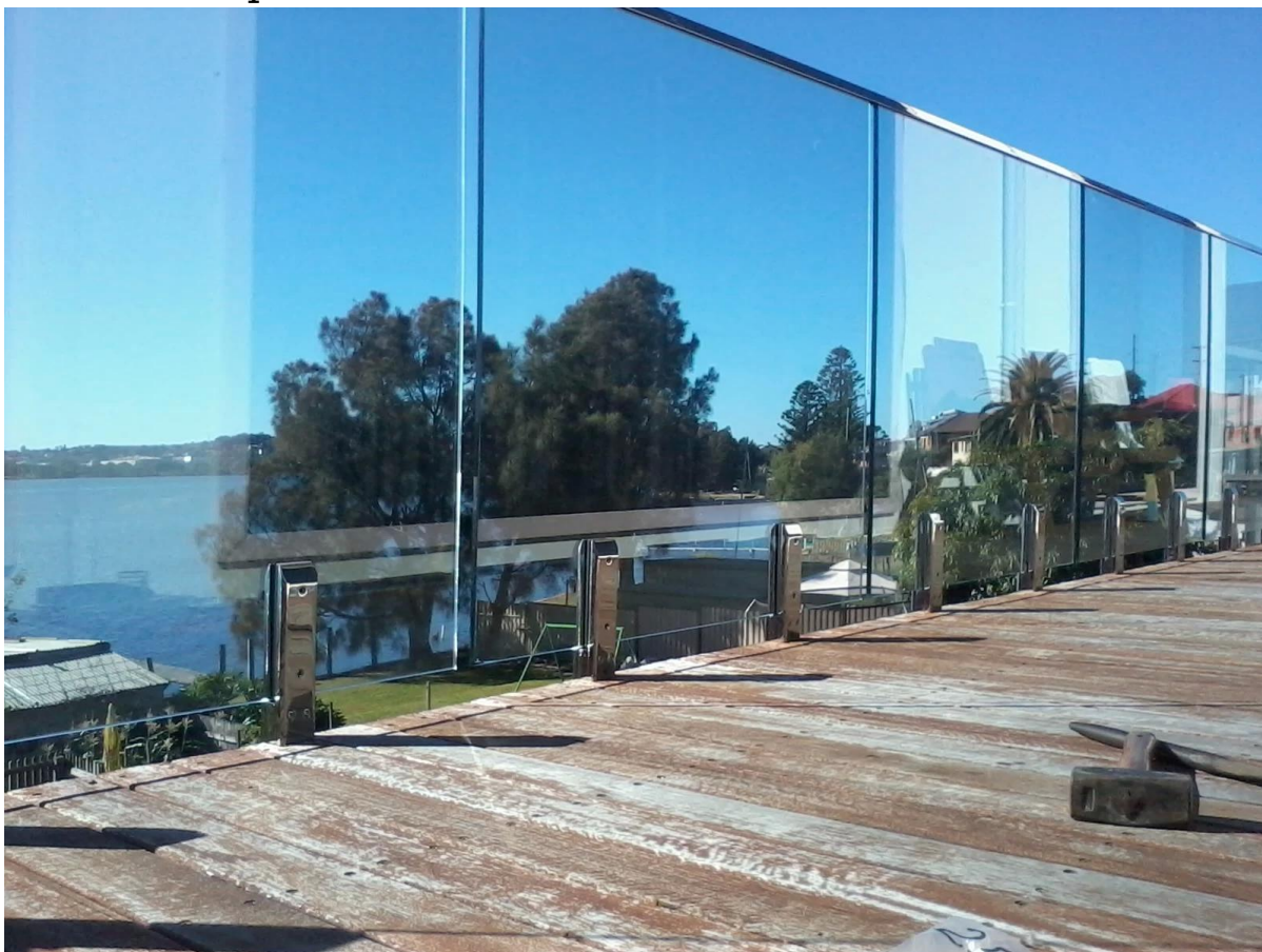
installation photos of slot handrails
