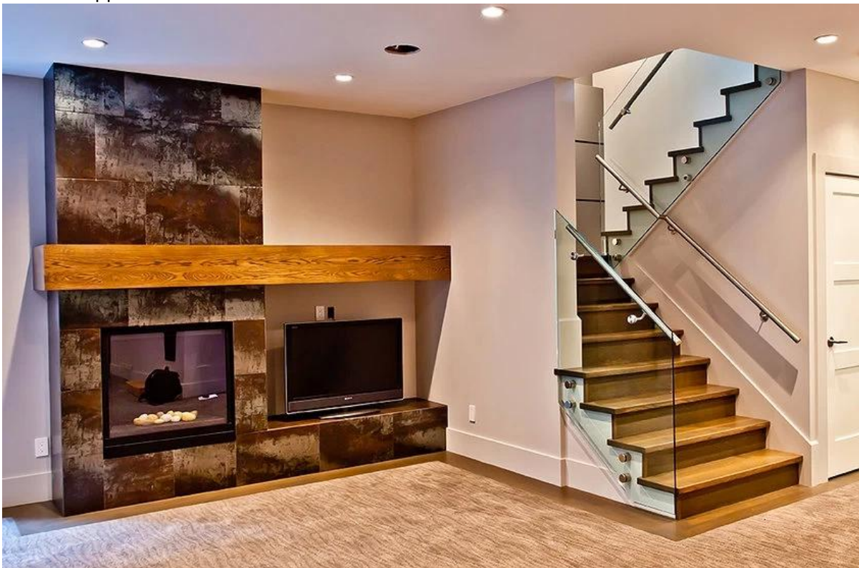
Standoff applied on indoor stairs :
