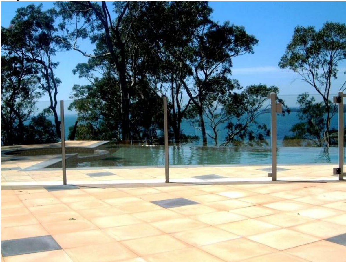
Glass balcony design 10-12mm tempered glass railing with aluminum post;
