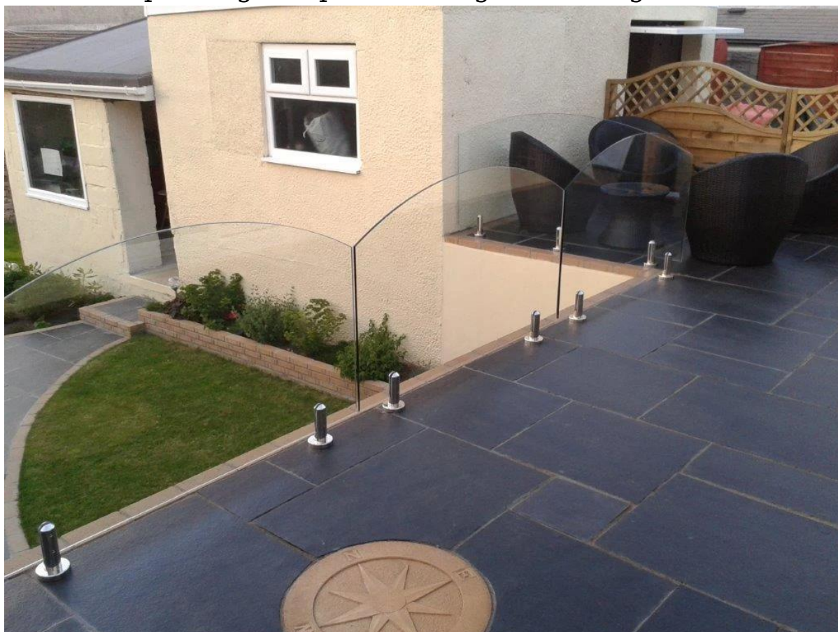
Clear tempered glass panels for glass railings-
