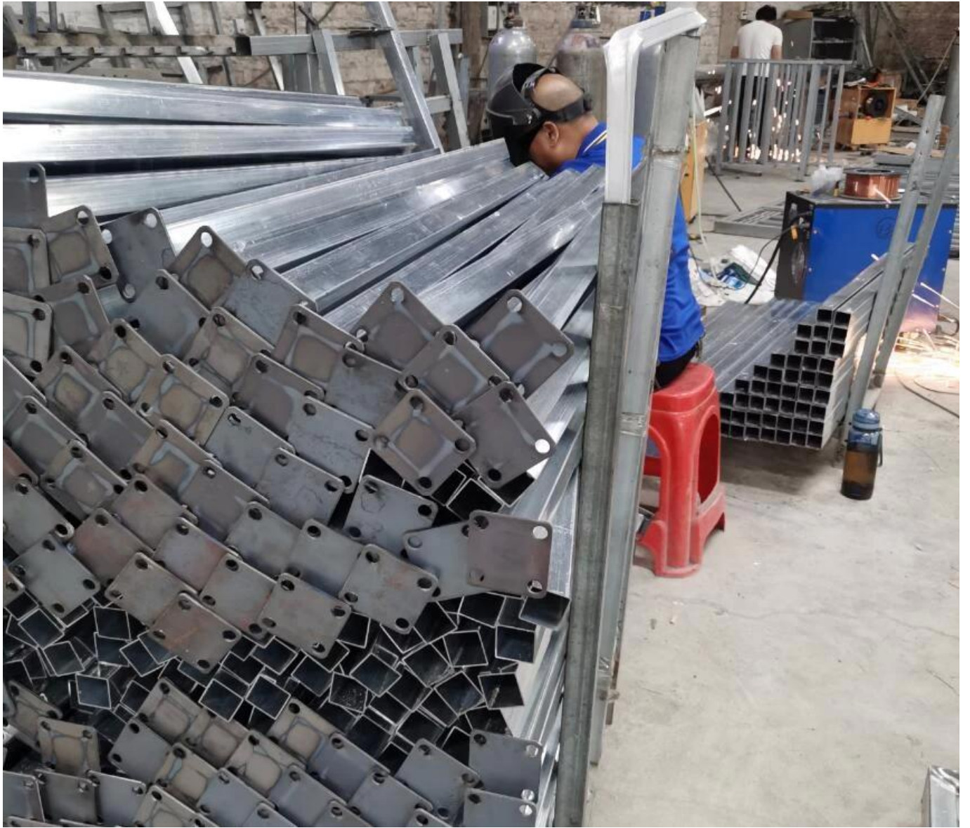
Powder coating of aluminum Railings-
