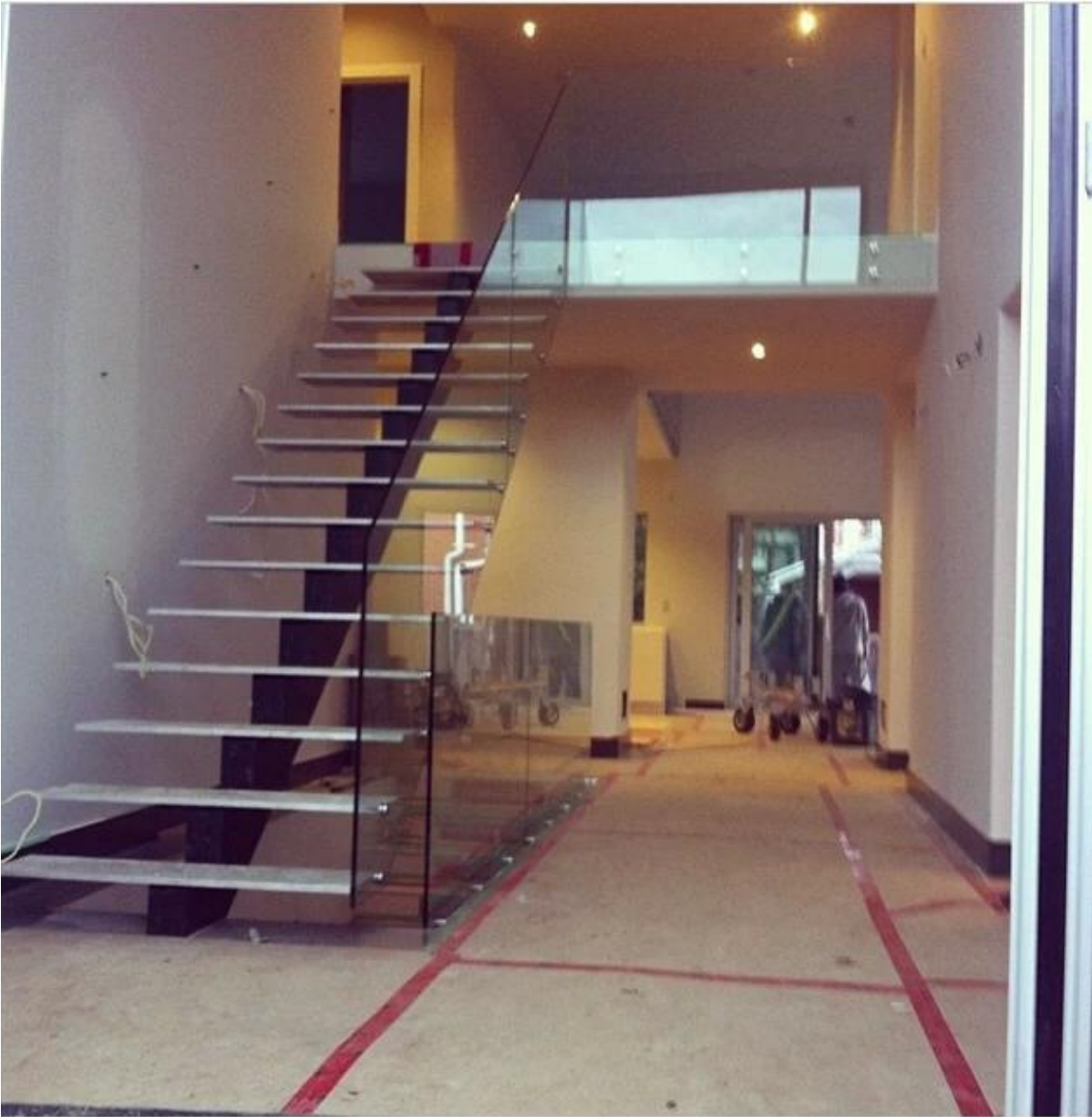
frameless glass railing work with stainless steel 316 glass standoff stand offs
