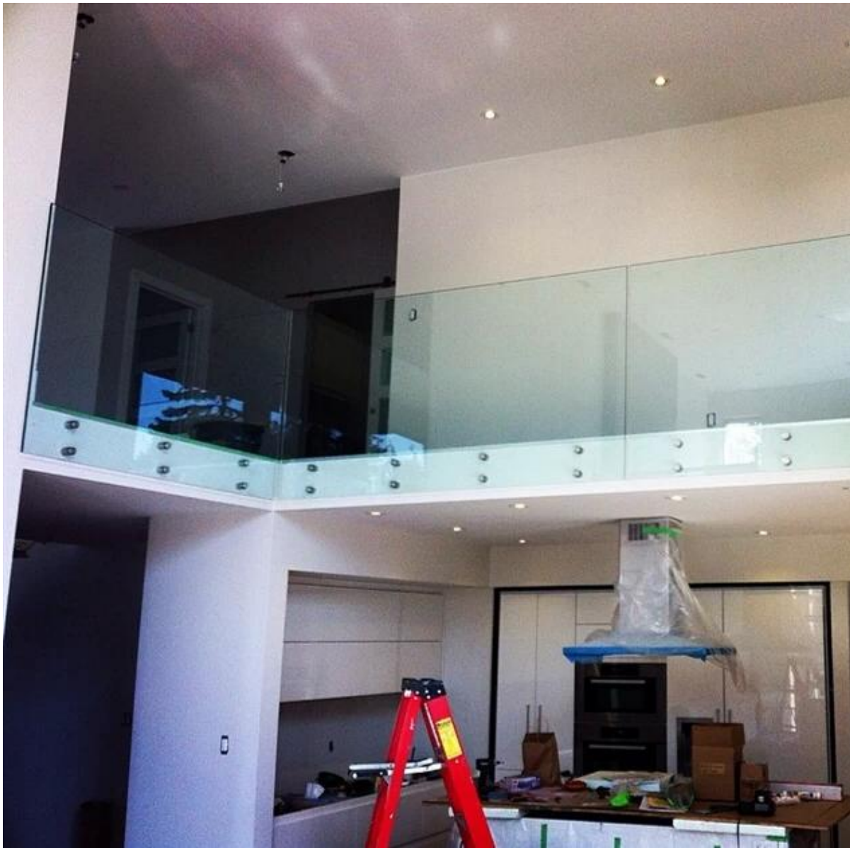
outdoor and indoor glass standoff, frameless standoff glass railing design, stainless steel glass standoff bracket
