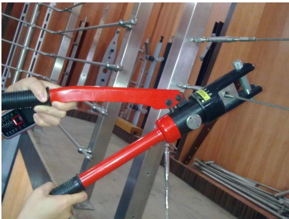
Cable tensioner installation
