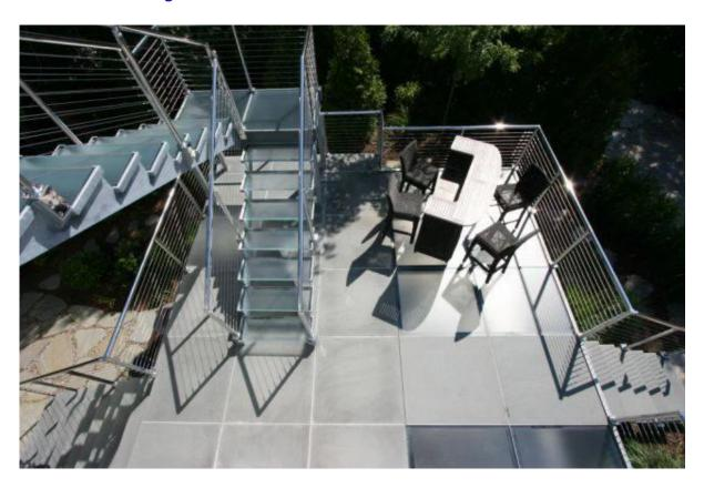
stainless steel wire rope railing system for outdoor balcony and staircase
