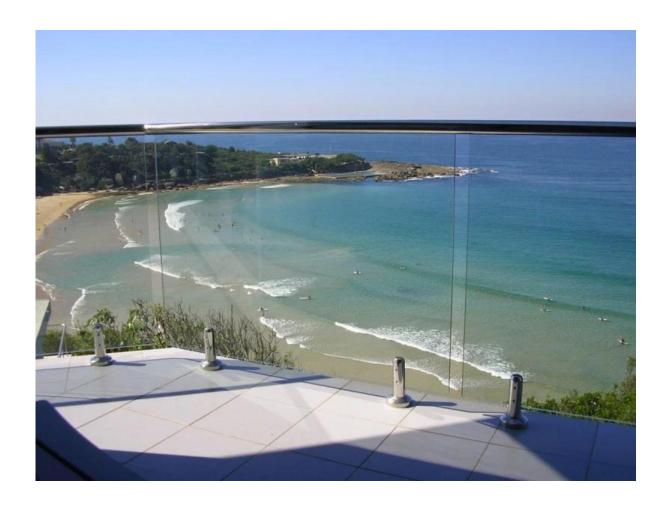
Glass spigot **SCM-2** -Net weight:1.66kg/piece -Hight: 285mm, 90mm fixing into ground
