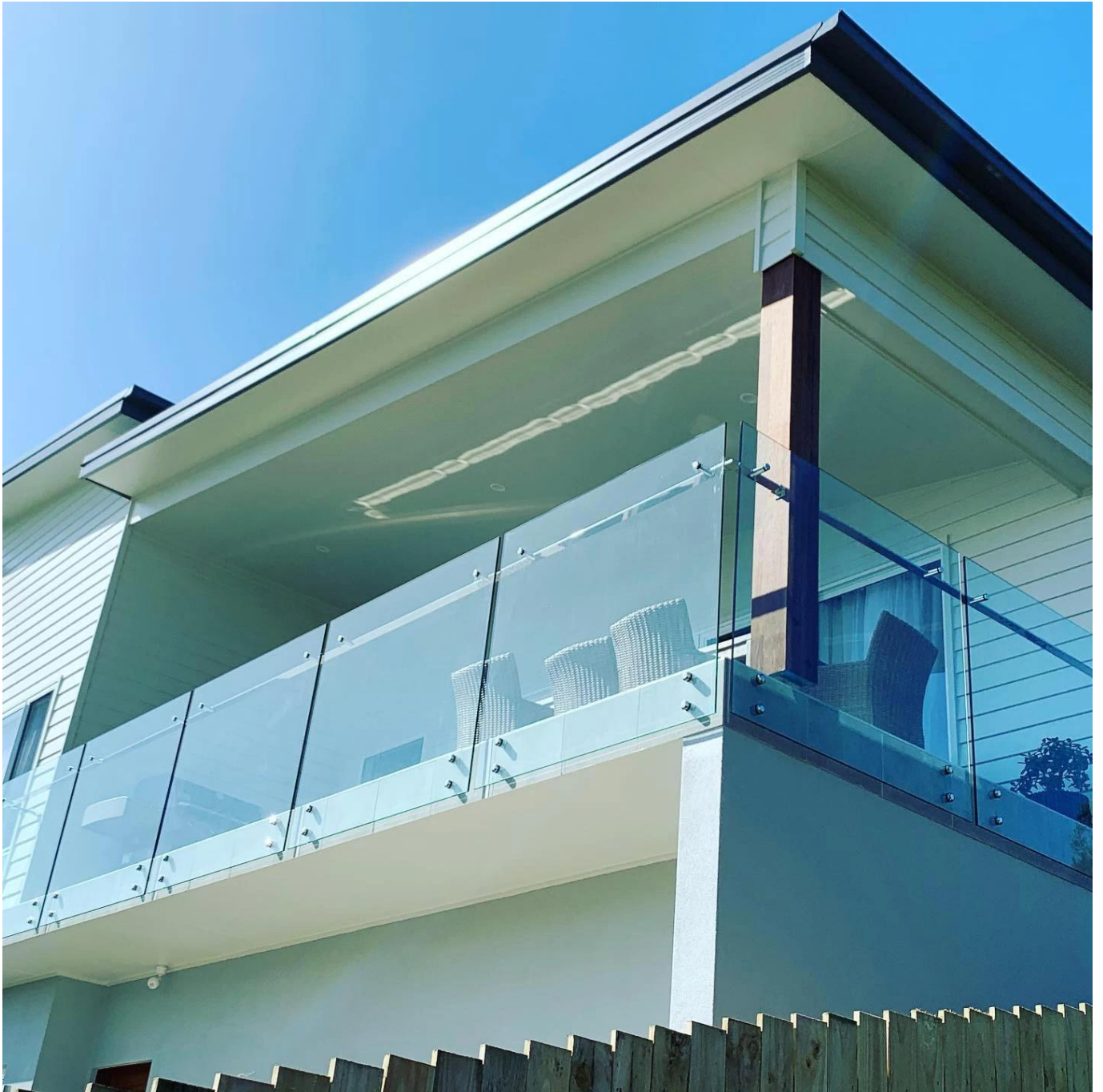
2) Glass standoff + glass clamp in between
